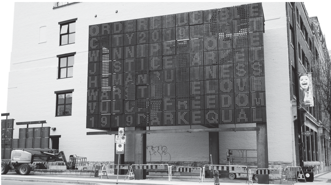
This large steel sign, unveiled at the corner of Lily and Market in 2017, is made of weathering steel. Shoe-horned into a small space between the sidewalk and the wall of a building, in a few short years it has become unintelligible to the viewer.
