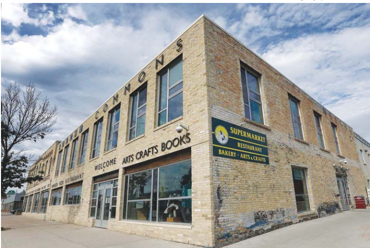
Neechi Commons is one of several community spaces which have closed recently.
